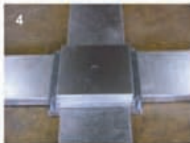
4 Fasten the trap frame, side blanks & ensure all the ductings and junction boxes are secured
