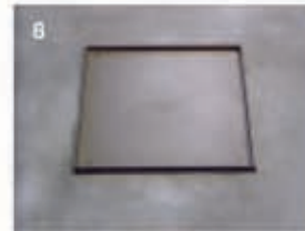
8 Finished installation without the carpet
