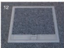
12 A finished floor with carpet
