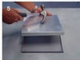
5 After screeding is cured, use a hammer & gently remove the disposable lid
