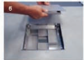
6 Remove the frame and trap by loosening the four corner
